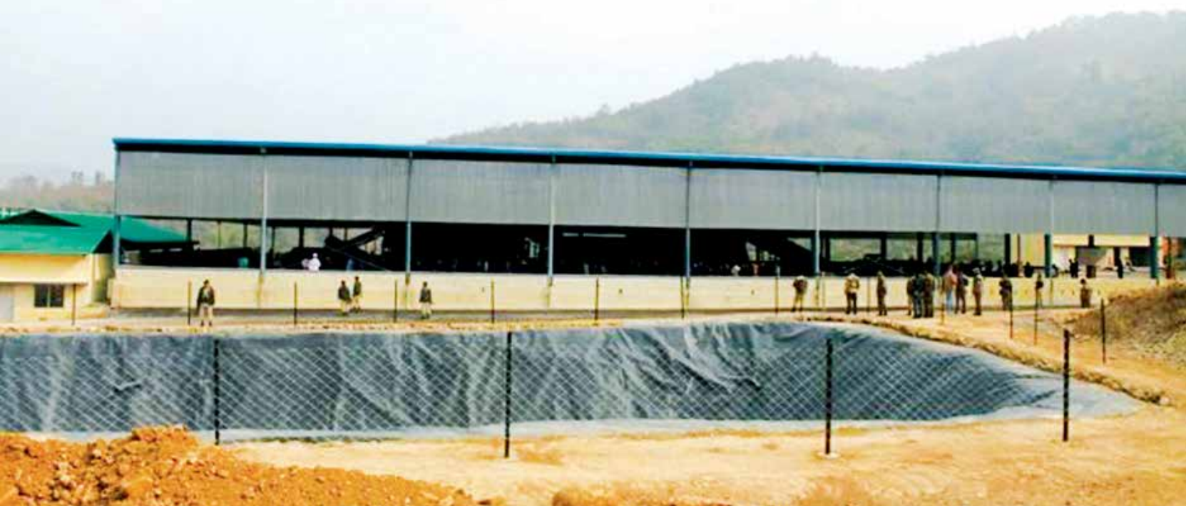
Solid Waste Disposal Plant at Kohima
